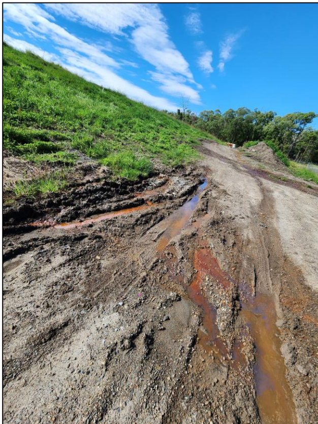
Figure 1: Potential leachate migrating from capped landfill area - south east of the leachate dam (8 April 2024)
