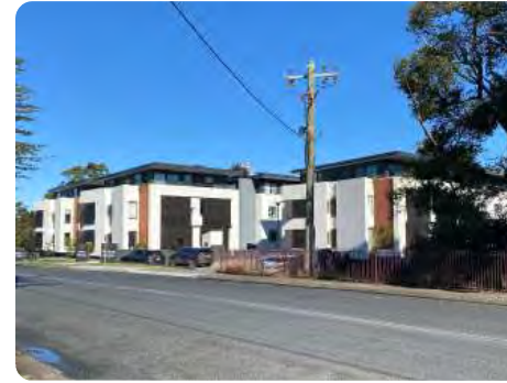
Figure 11: New medium density developments along Gregory Street are typically a maximum of three storeys
