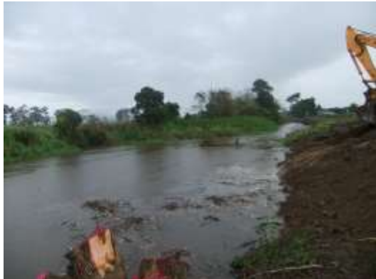
Figures 52 & 53: Show the earthen constriction and fallen Coral tree removed which has resulted in significant improvement to tidal flushing within the Upper Belmore River.
