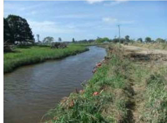
Figures 52 & 53: Show the earthen constriction and fallen Coral tree removed which has resulted in significant improvement to tidal flushing within the Upper Belmore River.
