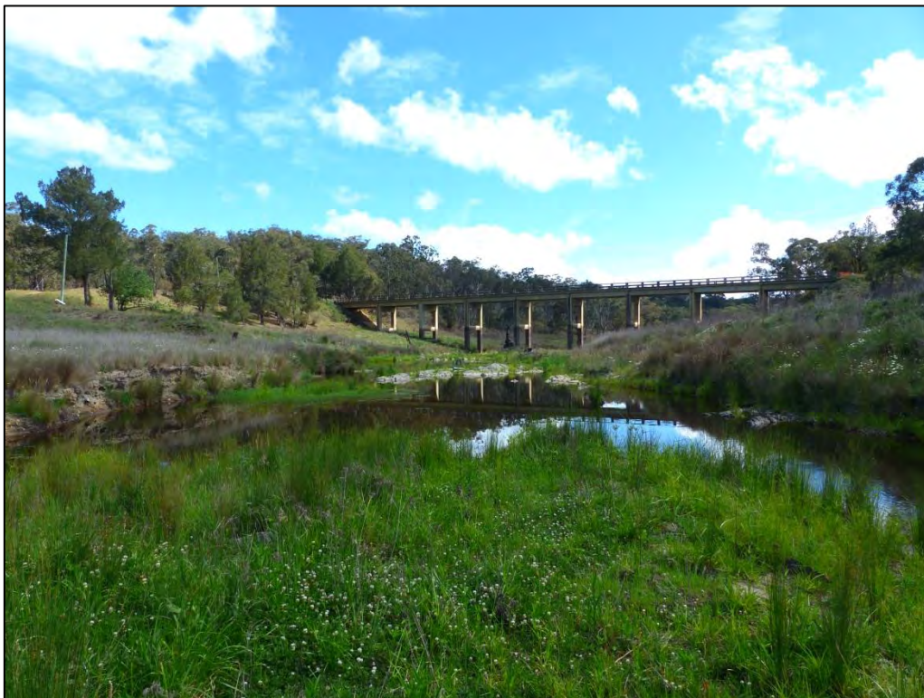
Plate 3.12 Site OAK1 on the Oaky River (looking downstream at the bridge on the Armidale-Kempsey Road).
