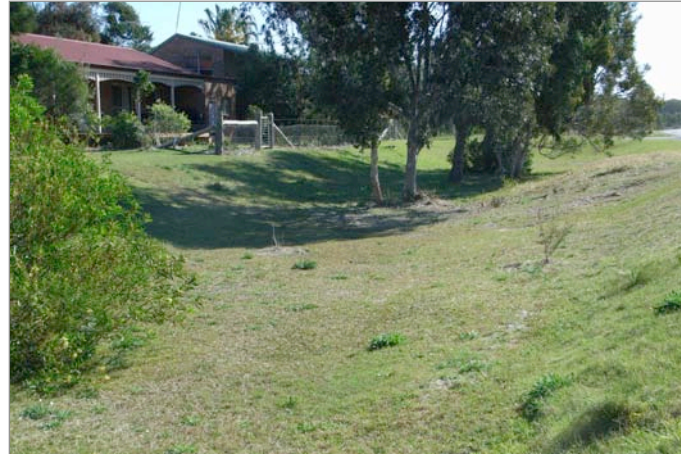
Plate 10 Swale drainage adjacent to Gap Road (Photo: Tim Ruge, GeoLINK)
