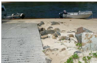
Plate 13 Hat Head boat ramp showing rocked abutments
