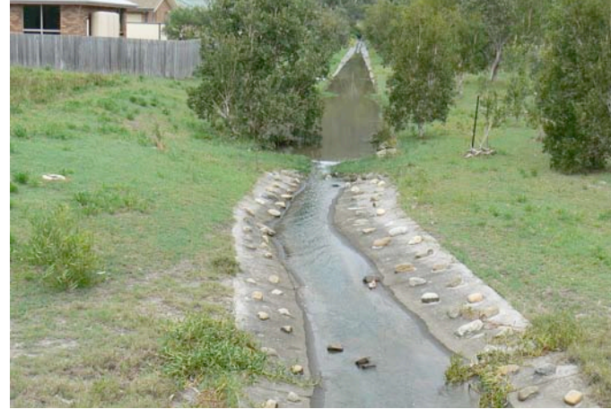
Plate 8 Hard channels deliver stormwater direct to the estuary without opportunity for filtering
