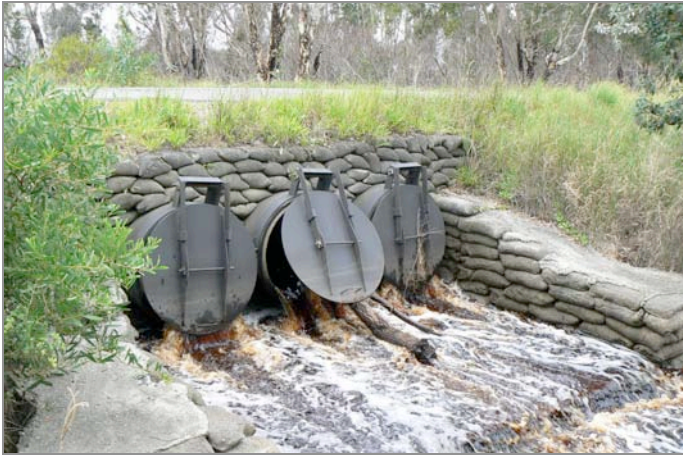
Plate 7 Floodgated stormwater drains
