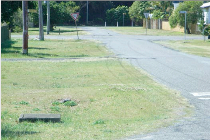
Plate 9 Swales provide improve filtering of stormwater before it enters the creek thus reducing pollutant loads (Photo: Tim Ruge, GeoLINK)
