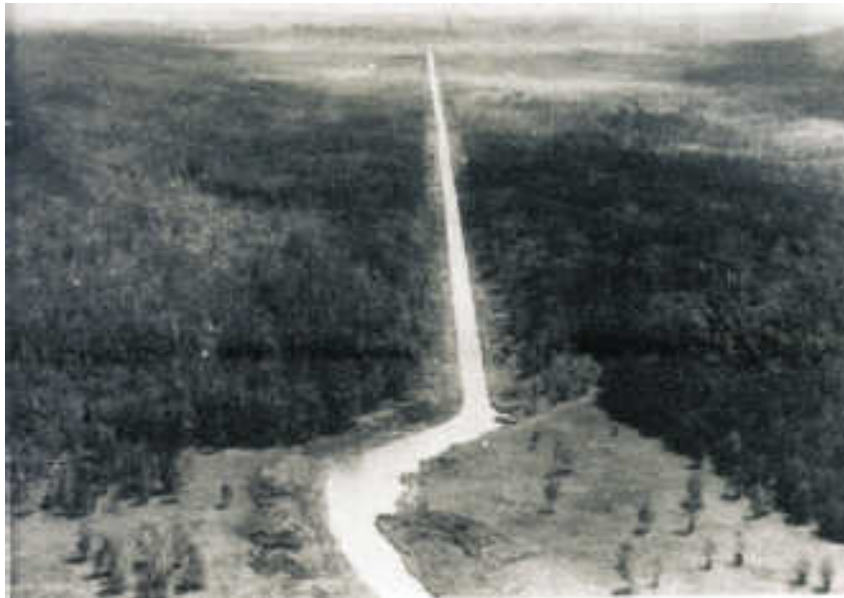
Aerial view of completed waterway
