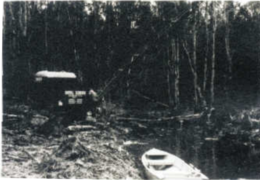
Clearing and excavating waterway through ti-tree jungle
