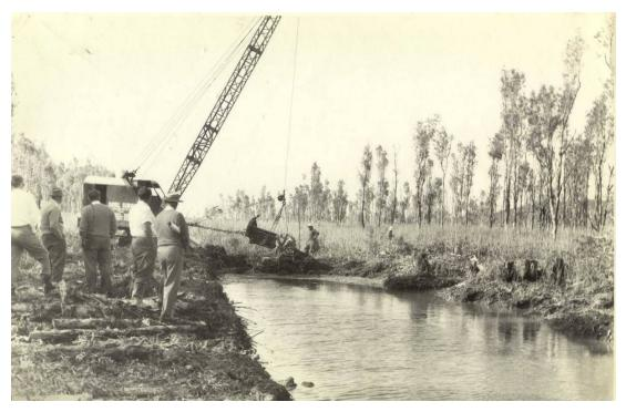
Figure 4-3 Excavation to create Killick Drain in the 1950s (photo courtesy KSC)
