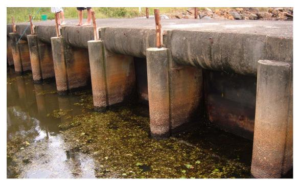
Figure 4-4 Killick Creek Floodgates and dropboards (submerged)
