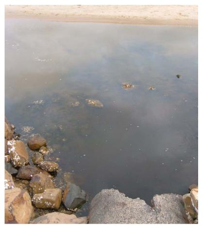
Figure 4-6 Rock apron formed from dislodged wall material
