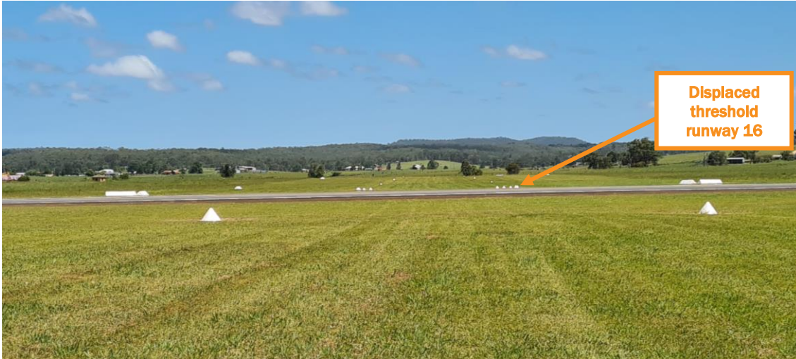
Figure 8 Close-up displaced threshold runway 16
