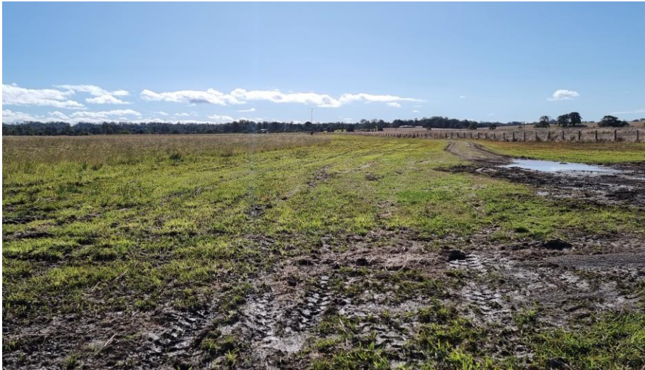
Figure 4. Waterlogged drainage areas south of the runway
