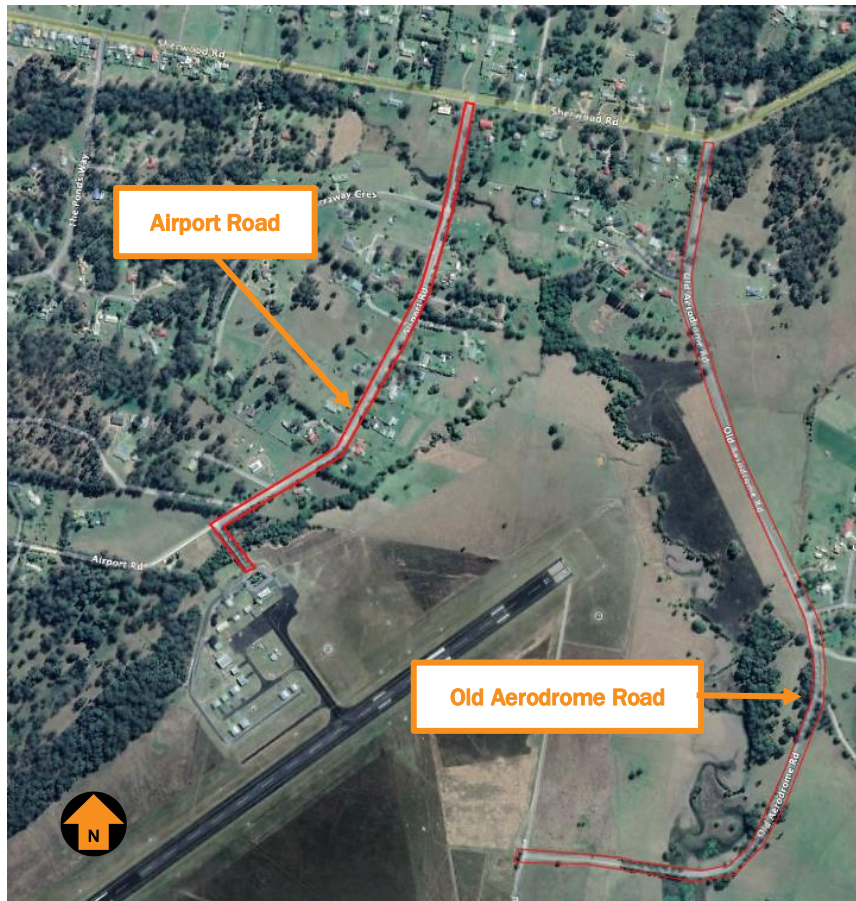
Figure 13. Entry roads to airport
