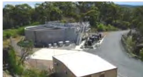
Amenities building & SBR tank
