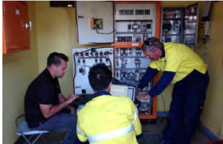
Trial testing of new radar SCADA system at Frederickton STP
