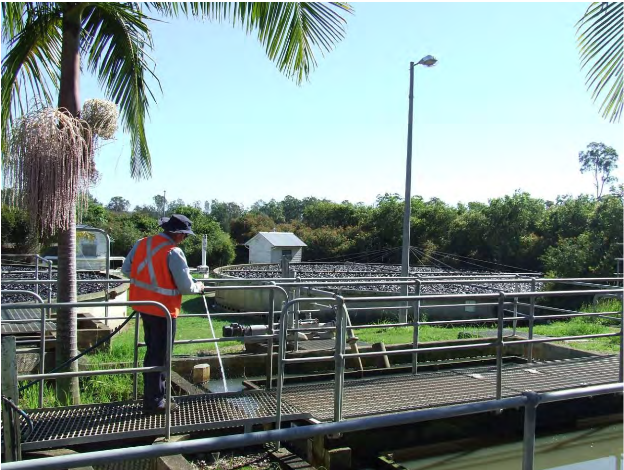
Cleaning the sedimentation tank at South Kempsey Sewer Treatment Plant
