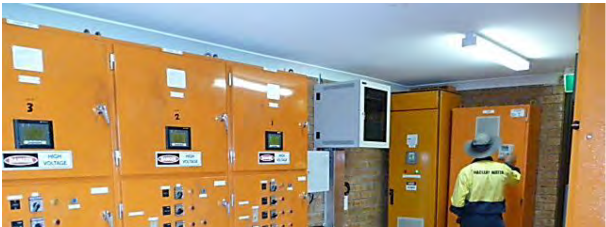
These switchboards & PLC run the pasveer channels at South West Rocks STP
