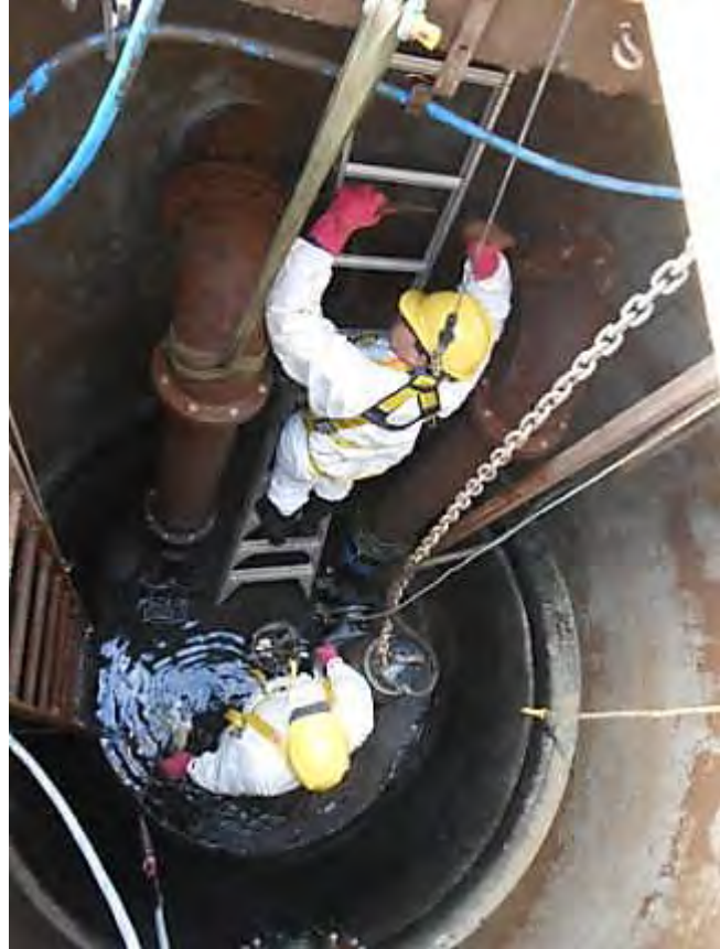
Mechanical fitters replacing discharge bends & rising main at K11B pump stn
