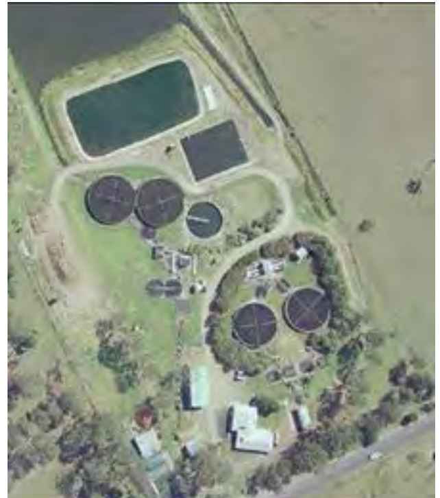
Aerial view of West Kempsey Sewer Treatment Plant
