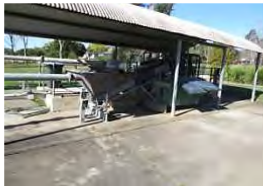
Amenities (above) & Inlet works (below)
