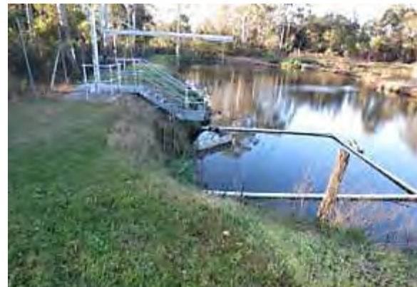
Lagoon monitoring platform
