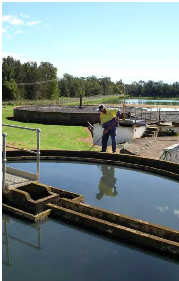
Sewer Process Operator attending to duties at West Kempsey STP
