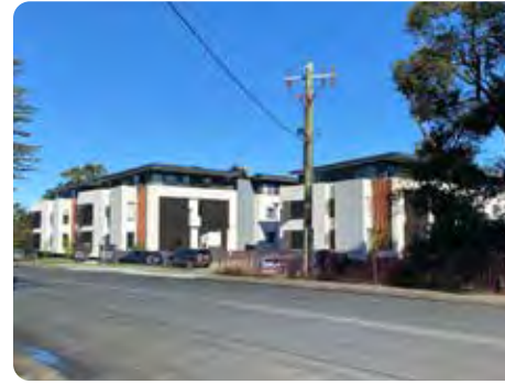
Figure 11: New medium density developments along Gregory Street are typically a maximum of three storeys
