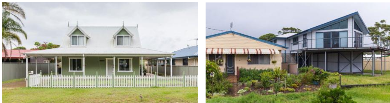
Existing housing, Stuarts Point
