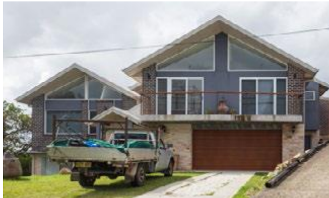
Existing Housing, Crescent Head
