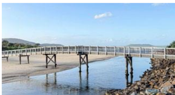
Crescent Head (Killick Creek) Foot Bridge
