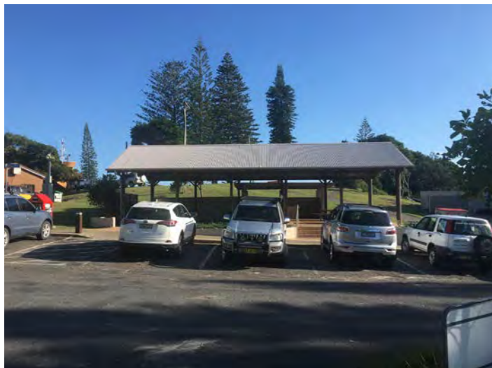
Access and safety issues resulting from incompatible adjacent uses
