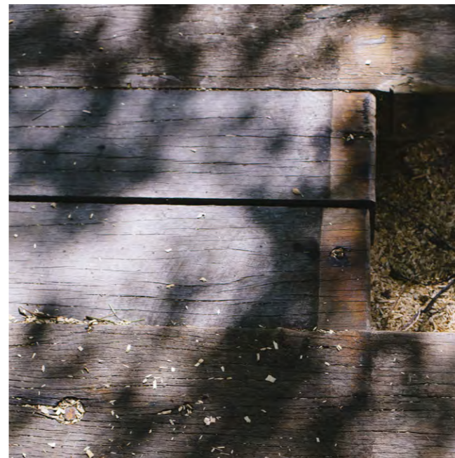
Custom timber elements- utilizing KSC recycled bridge timbers where appropriate
