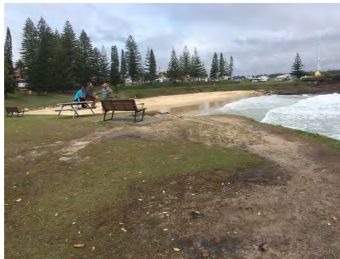
Erosion along the informal path areas and adhoc furniture placement and style
