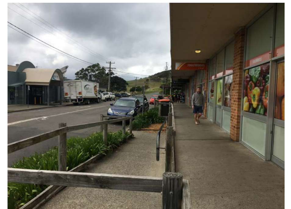
Existing accessible ramps on Rankine Street- poor quality access and amenity. Reduces footpath width in a critical circulation zone
