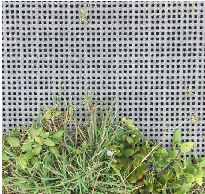
Example of mesh material installed at grade to allow vegetation to blur the edges
