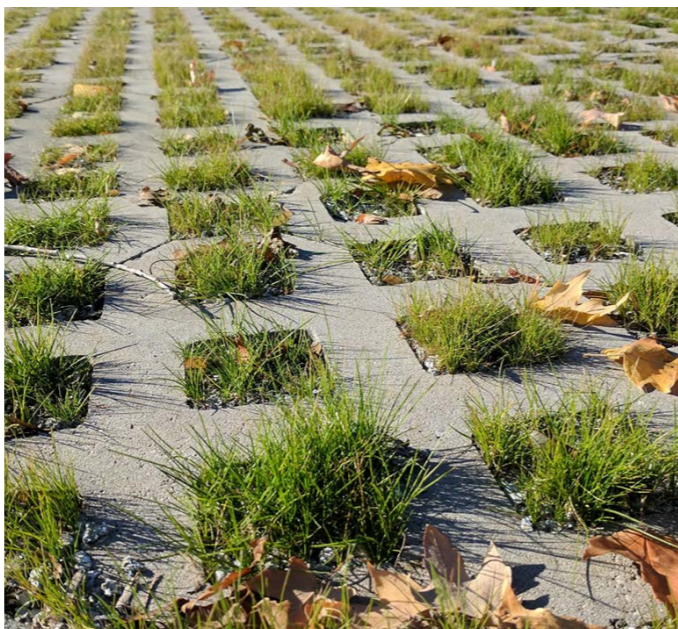
Permeable paving example- boat ramp access and associated parking
