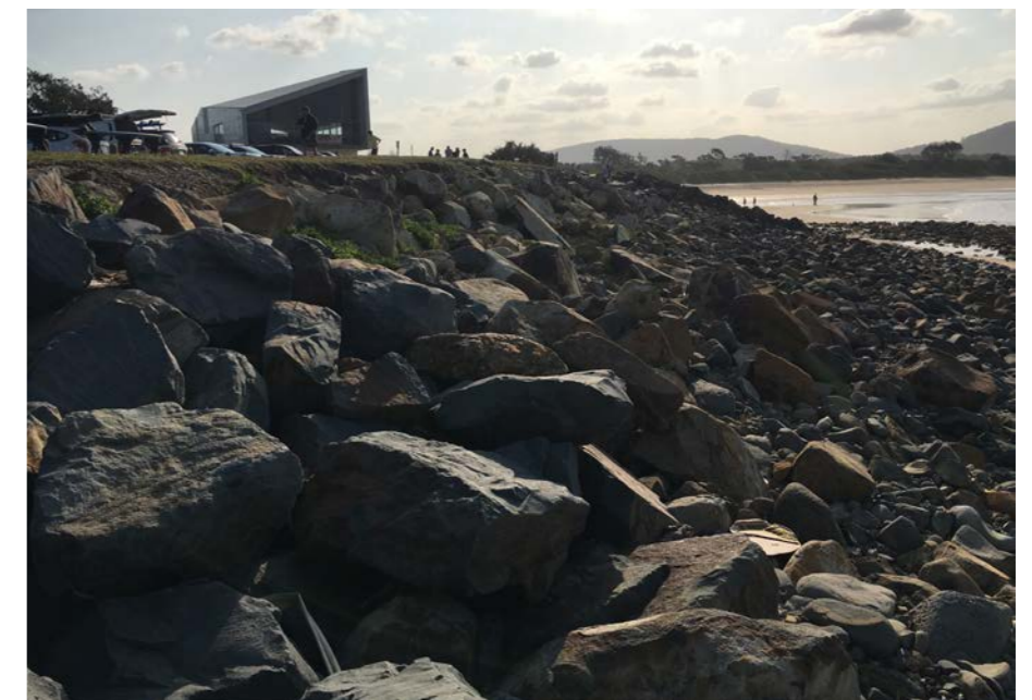
Existing erosion protection measures
