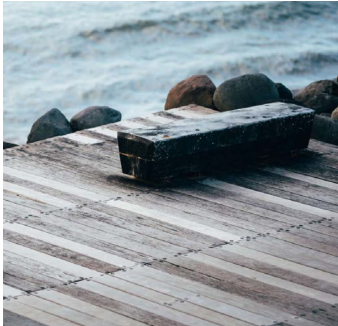
Timber deck and timber bench seats- complimentary material relationship with stone
