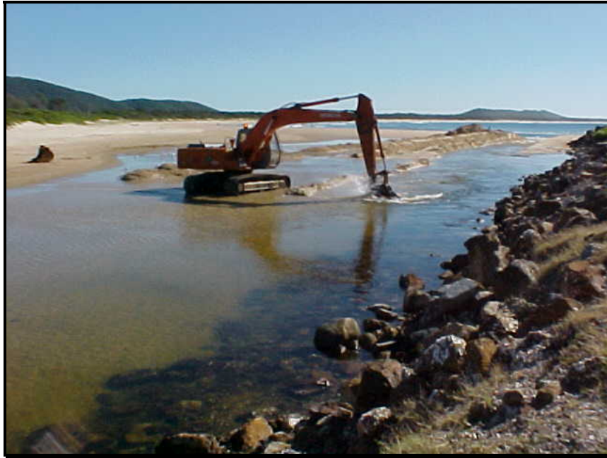
Figure A1 Artificial Entrance Opening of Killick Creek: April 2004
