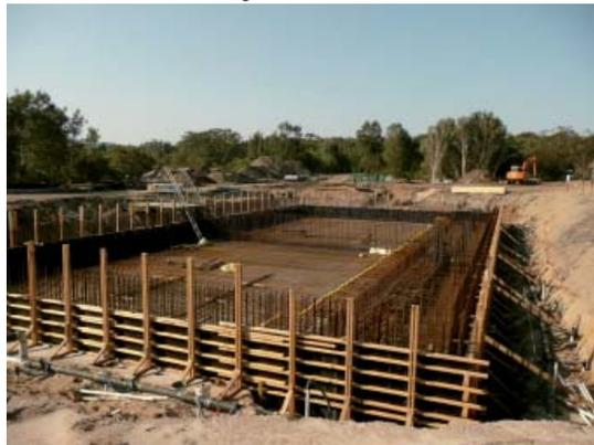
shows progress on concrete works for the sequence batch reactor (SBR), which is the main process component of the new plant.
