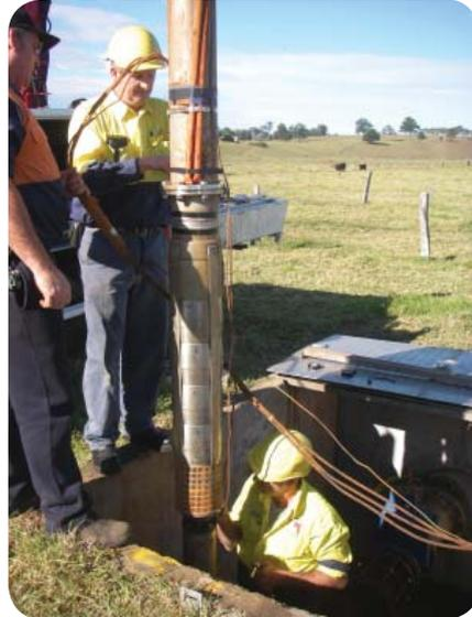
Above: (Left) The bore column is lifted so the pump can be removed and (on the right) Macleay Water staff re-position the pump in the bore hole after the maintenance work is completed.
