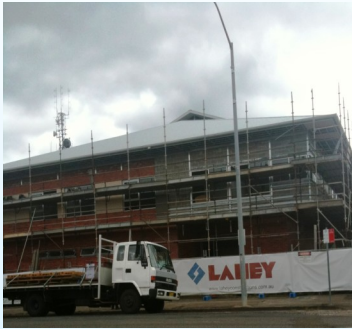
Construction of new Police Station
