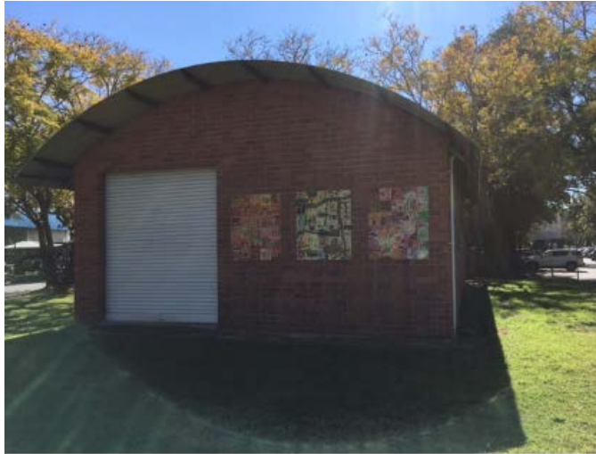
Photo 4 – Space adjacent to the Existing Shed Kempsey/Crescent Head Boat Storage Shed
