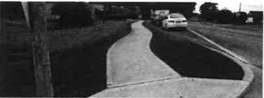
Steve Eggleton Drive PAMP works are nearing completion
