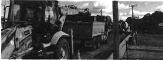
Kerb rehabilitation on Clarence Ryan Avenue, West Kempsey
