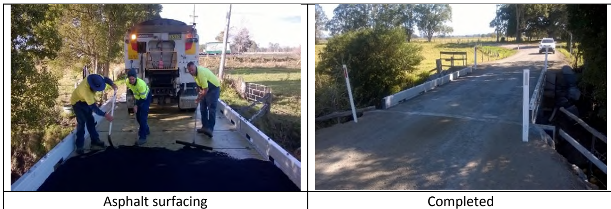
Placing composite fibre deck
